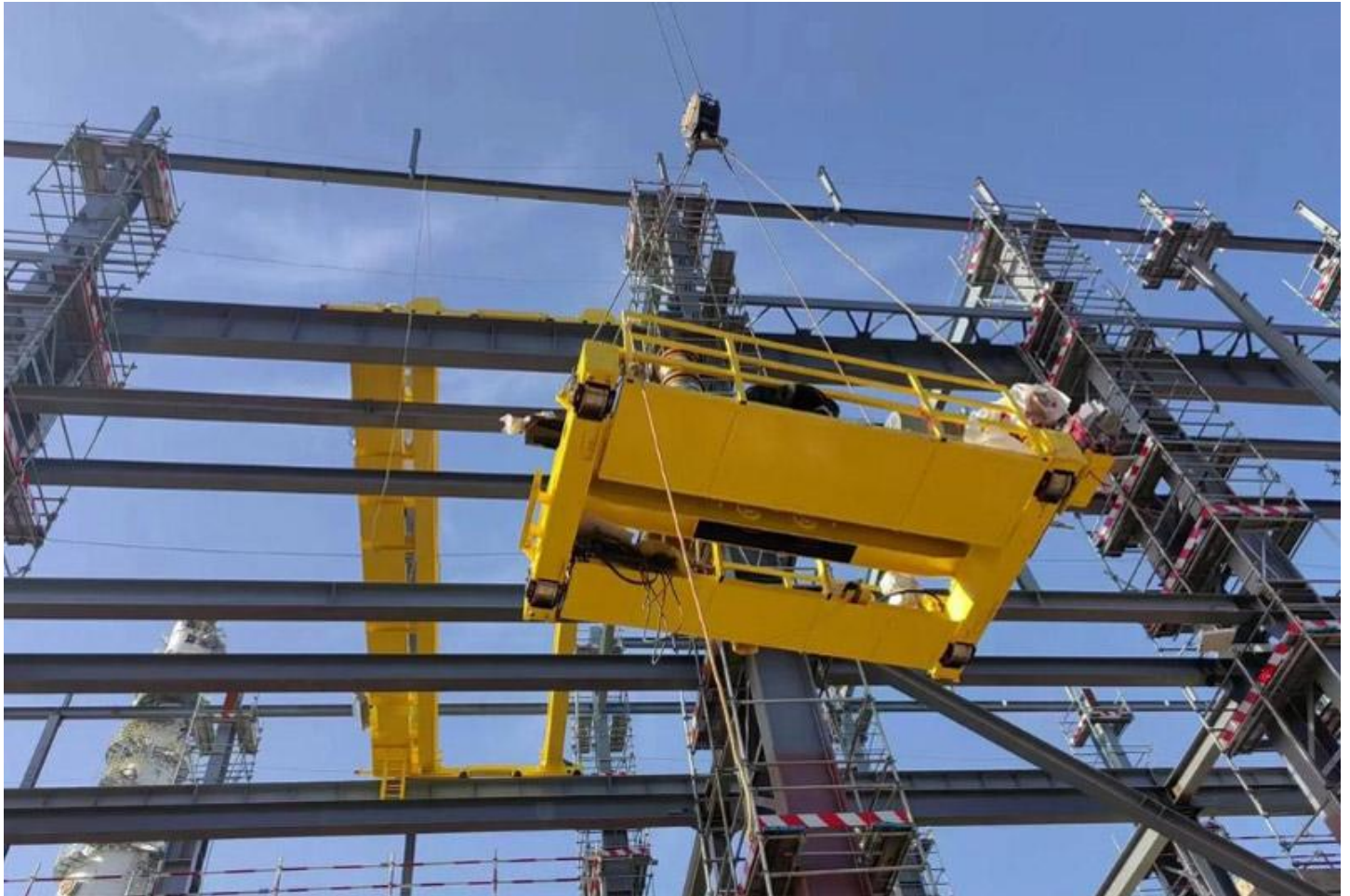
25-ton explosion-proof double girder overhead crane installation
