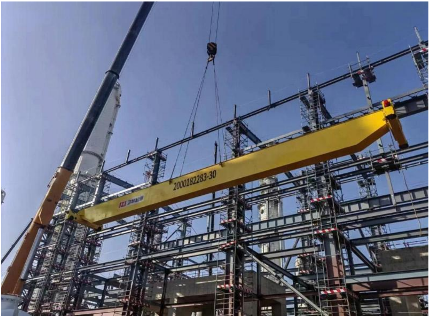
25-ton explosion-proof double girder overhead crane installation
