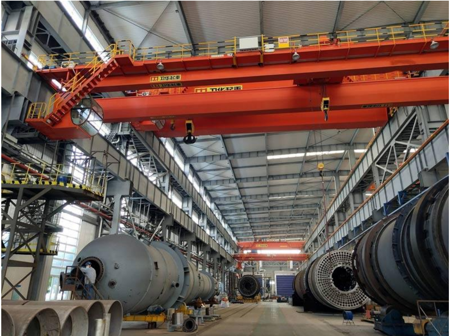
50 tons double girder overhead crane
